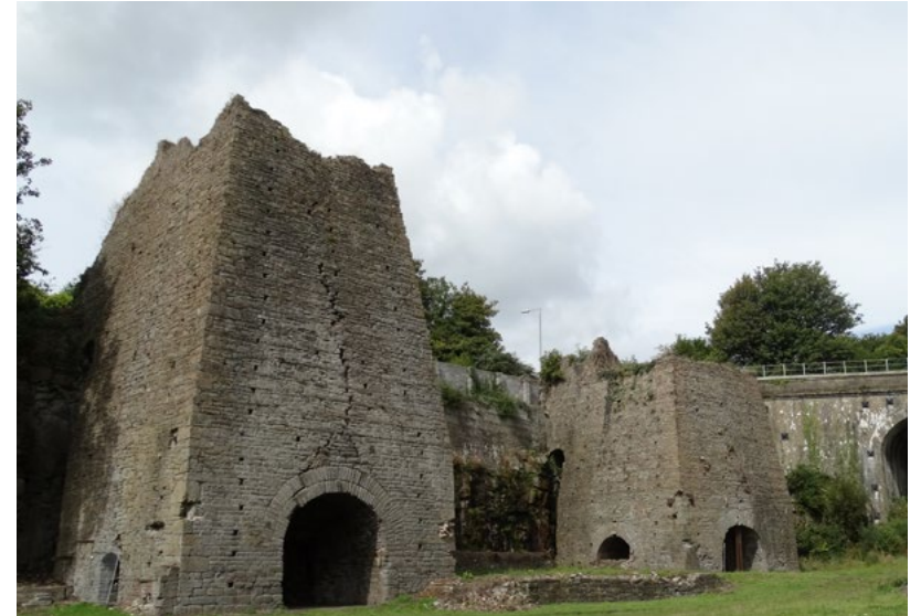
The work of dedicated volunteers who cleared vegetation from the Blast Furnaces at Neath Abbey Ironworks.
