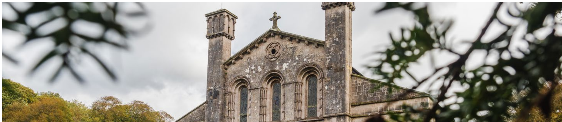
St Mary's Abbey Church, Margam (Grade I Listed Building).
