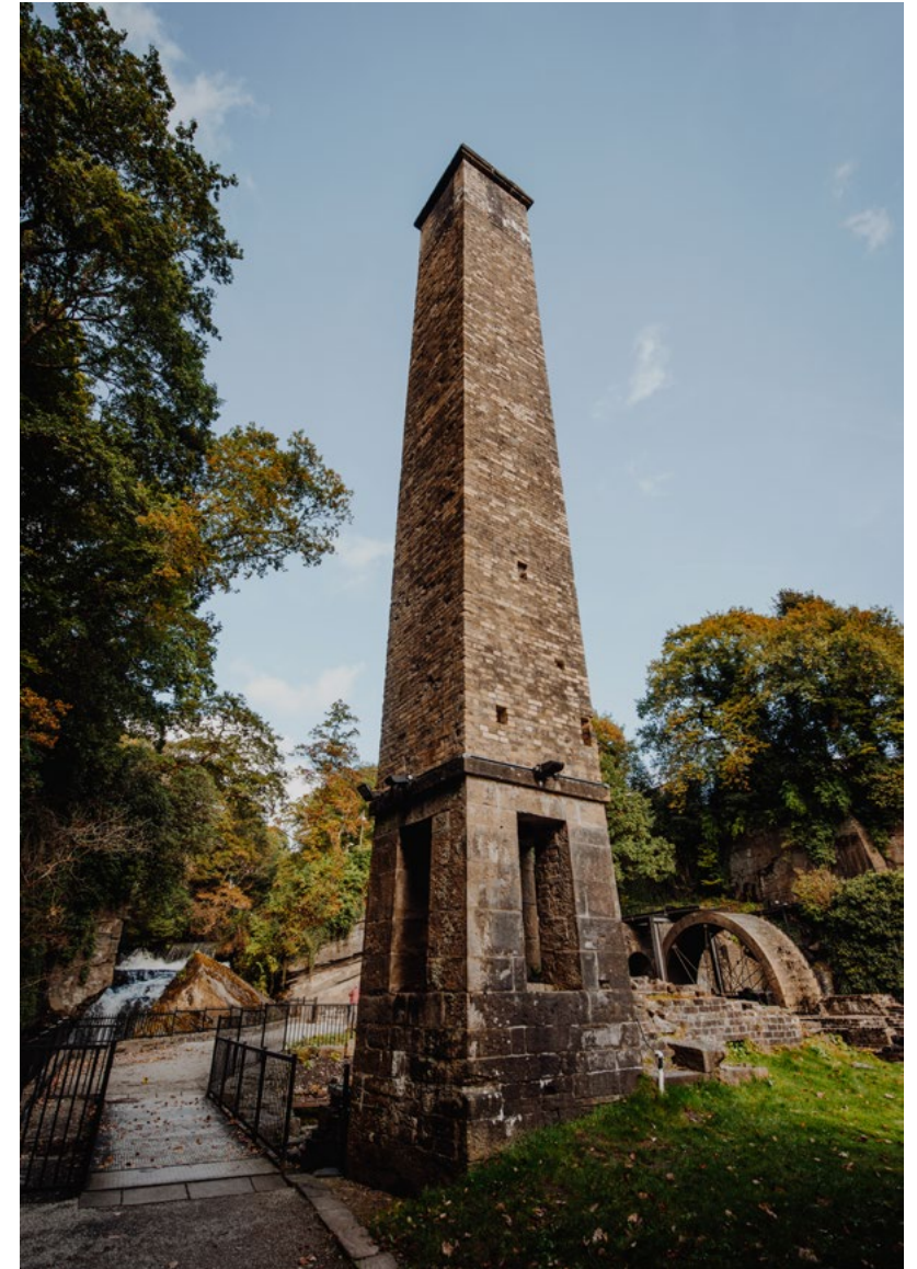
Chimney at Aberdulais Falls Tinplate Works (Grade II Listed Building).
